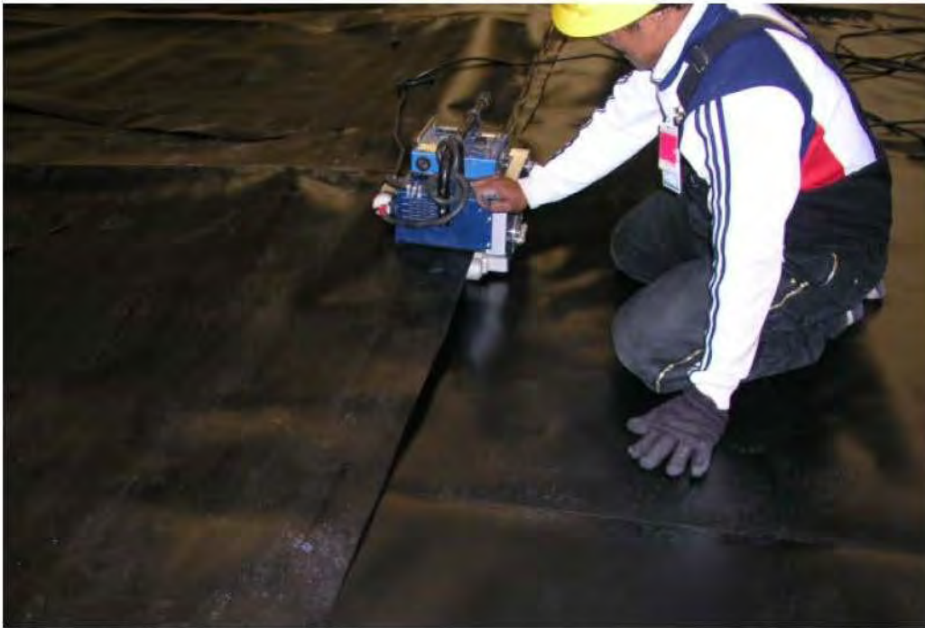
Photo 2-22 Welding of Geomembrane
