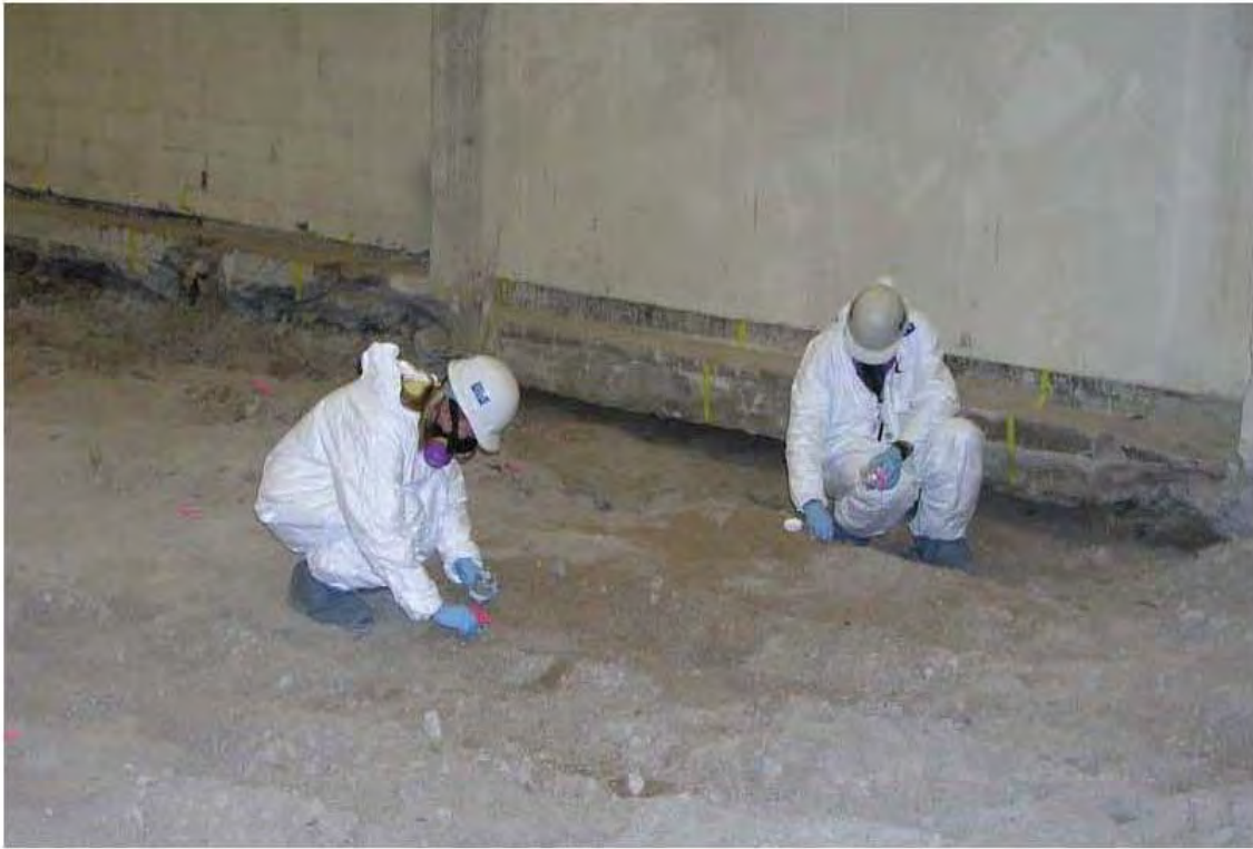
Figure 5.73 Sampling of Soil Subgrade Prior to Import of Granular Subgrade
