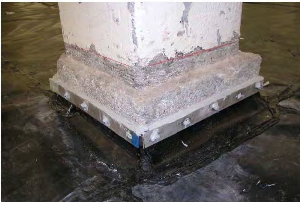
Photo 2-23 Geomembrane Detail Around Columns
