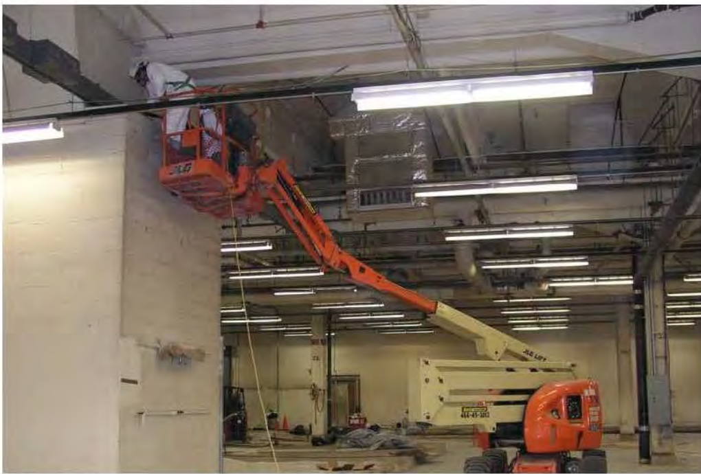
Photo 2-35 Cleaning of Walls and Overhead Piping/Surfaces
