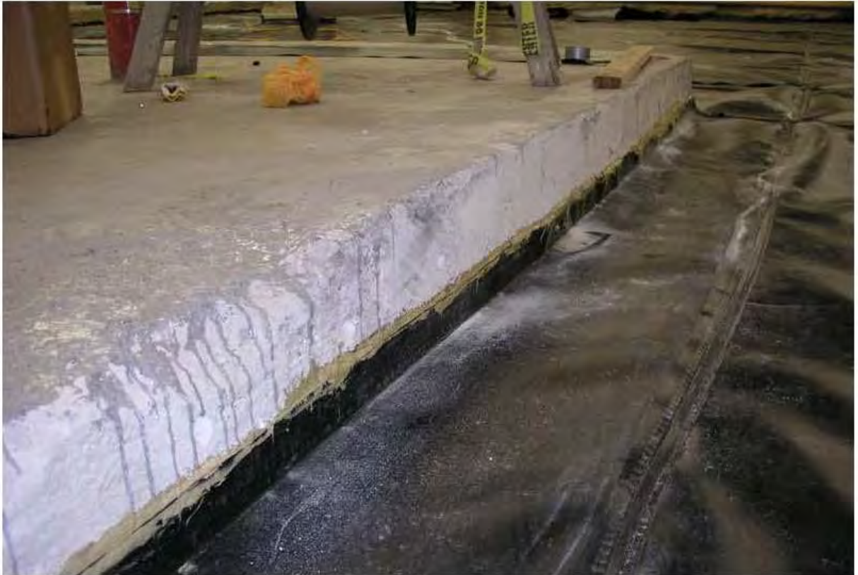
Photo 2-24 Geomembrane Detail at Basement Edge
