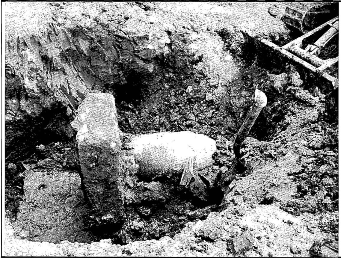
Figure 5.61 Column Footing and 4" Abandoned Line (Area B)
