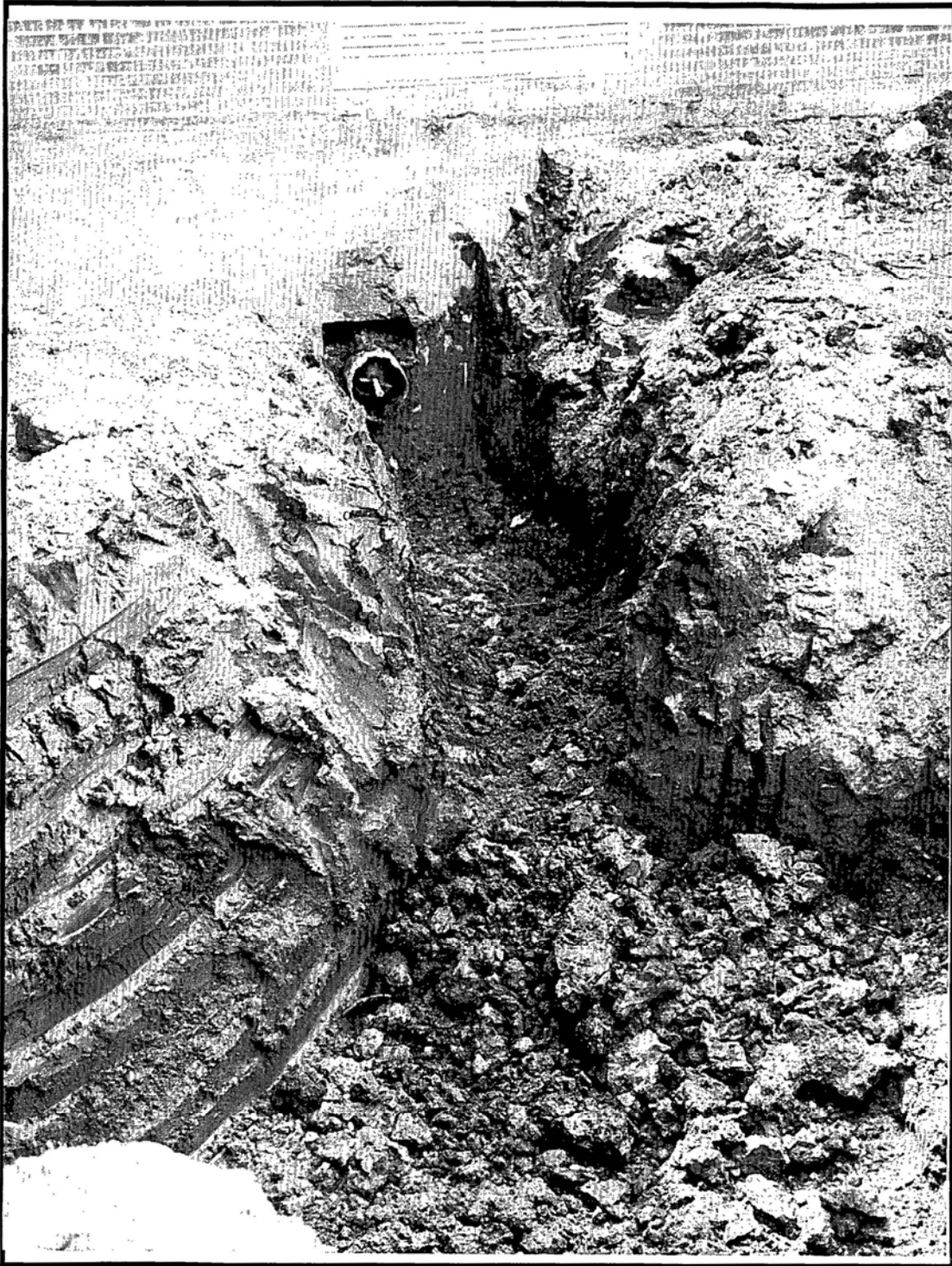
Figure 5.60 12" Sanitary Line Removed and Plugged at MVB
