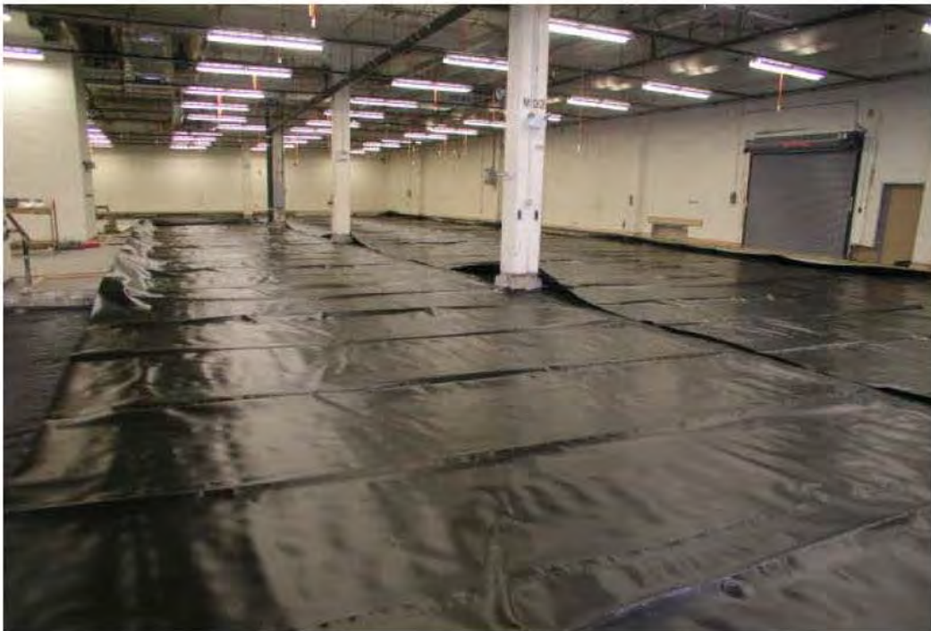
Photo 2-21 Placement of 40-mil Geomembrane
