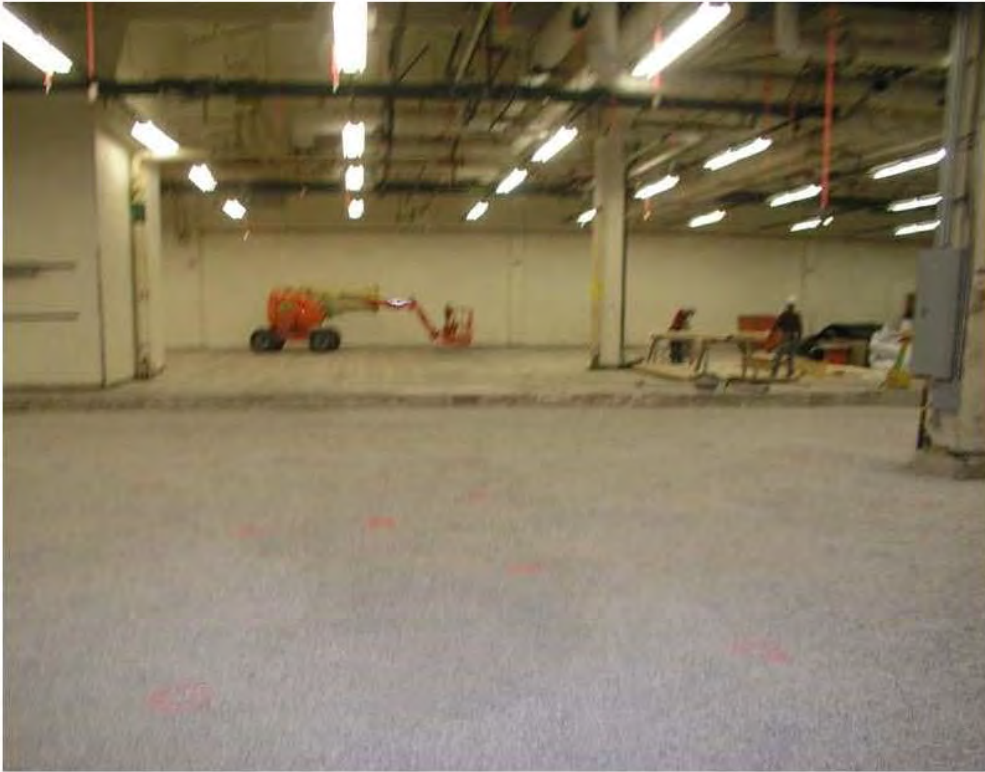
Photo 2-18 New Aggregate Base
