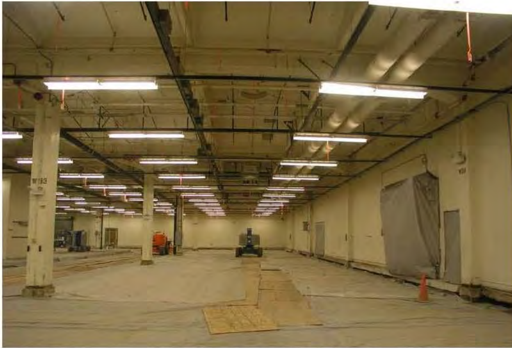
Photo 2-36 Post Cleaning Confirmation Sampling of Overhead Surfaces
