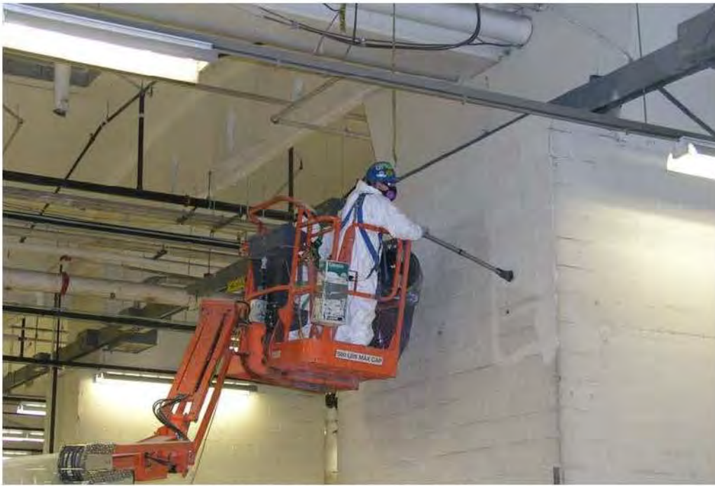
Photo 2-34 Cleaning of Walls and Overhead Piping/Surfaces
