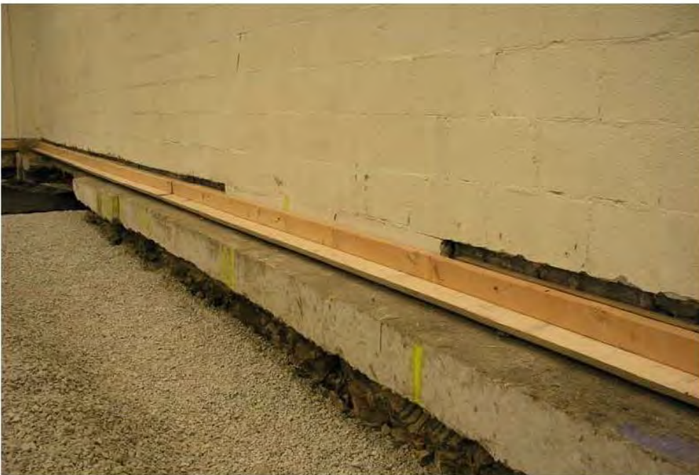
Photo 2-19 New Aggregate Base and Wall Edge Detail
