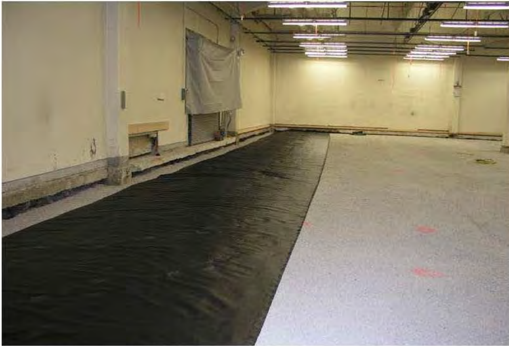
Photo 2-20 Placement of 20-mil Geotextile Cushion
