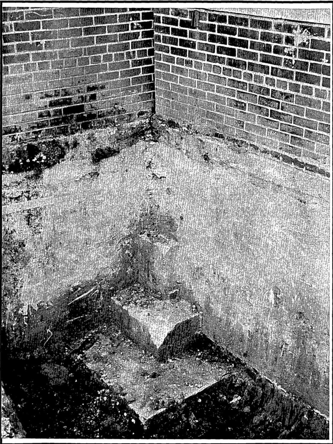
Figure 5.62 Bottom of Area A with MVB Footing
